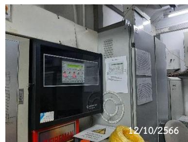
Fire Alarm Control Panel
