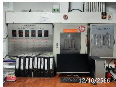
Graphic Annunciator Fire Alarm System
